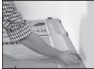
Centre/angle the installation area and adjust the first row of planks by cutting it to size.
