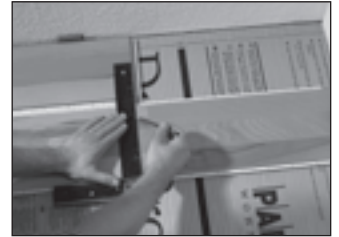
Cut the last plank of the first row to the necessary length, considering the wall clearance. The cut piece of the plank is used to start the second row.
