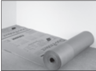
Lay the underlay on the prepared subfloor.
