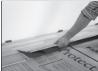
Start the next row from the left. Simply click the long sides of the planks together. The planks must not be glued.
