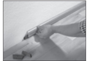
Cover edge clearances using matching skirting boards from the extensive Parador product range.
